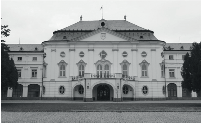
Figure 2. The former Episcopal Summer Palace
